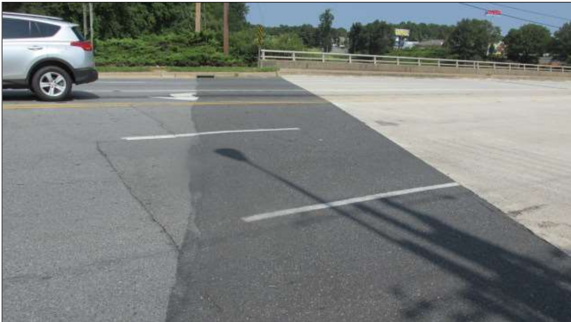
THE APPROACHES PATCHED IN PAST FULL WIDTH X 15' LONG.
