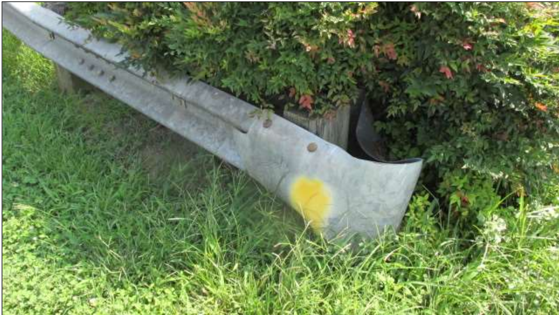
GUARDRAIL END FOR THE NORTHEAST AND SOUTHWEST CORNERS
