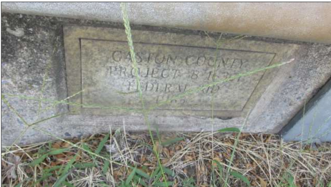
INFOR. PLATE AT THE NORTHEAST CORNER
