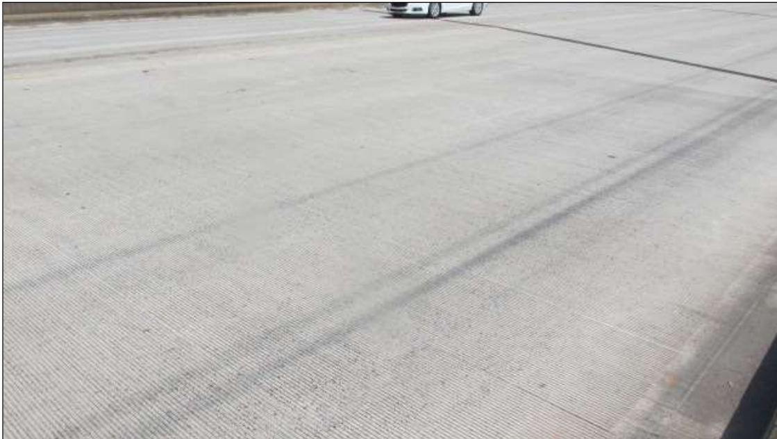
DECK REHABED SINCE LAST INSP.
