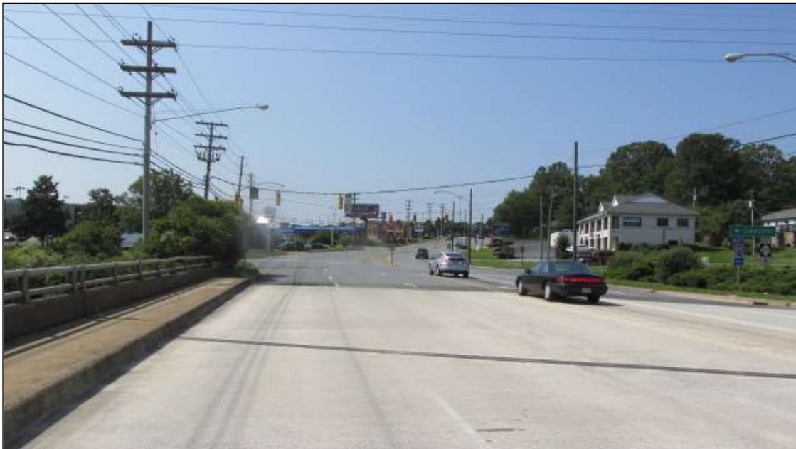
GUARDRAIL LOOKING EAST
