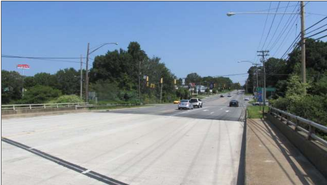
GUARDRAIL LOOKING WEST
