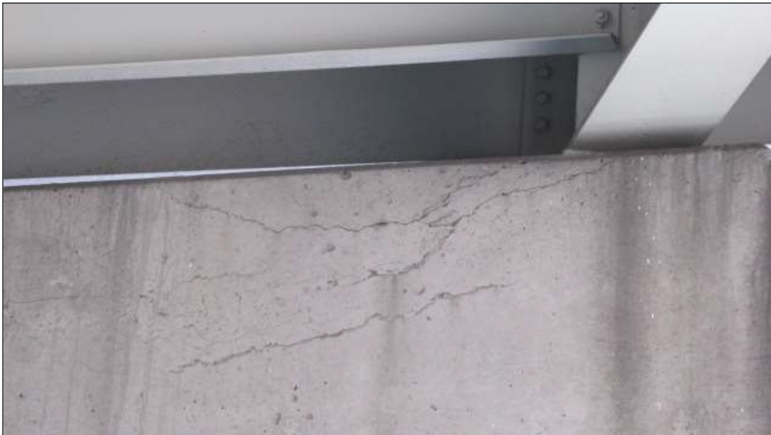
CRACKING ALONG THE SOUTH FACE OF BENT 3 UNDER BEAM. 4.
