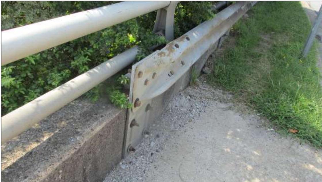
GUARDRAIL ATTACHED TO THE BRIDGE RAIL FOR THE SOUTHEAST AND NORTHWEST CORNERS
