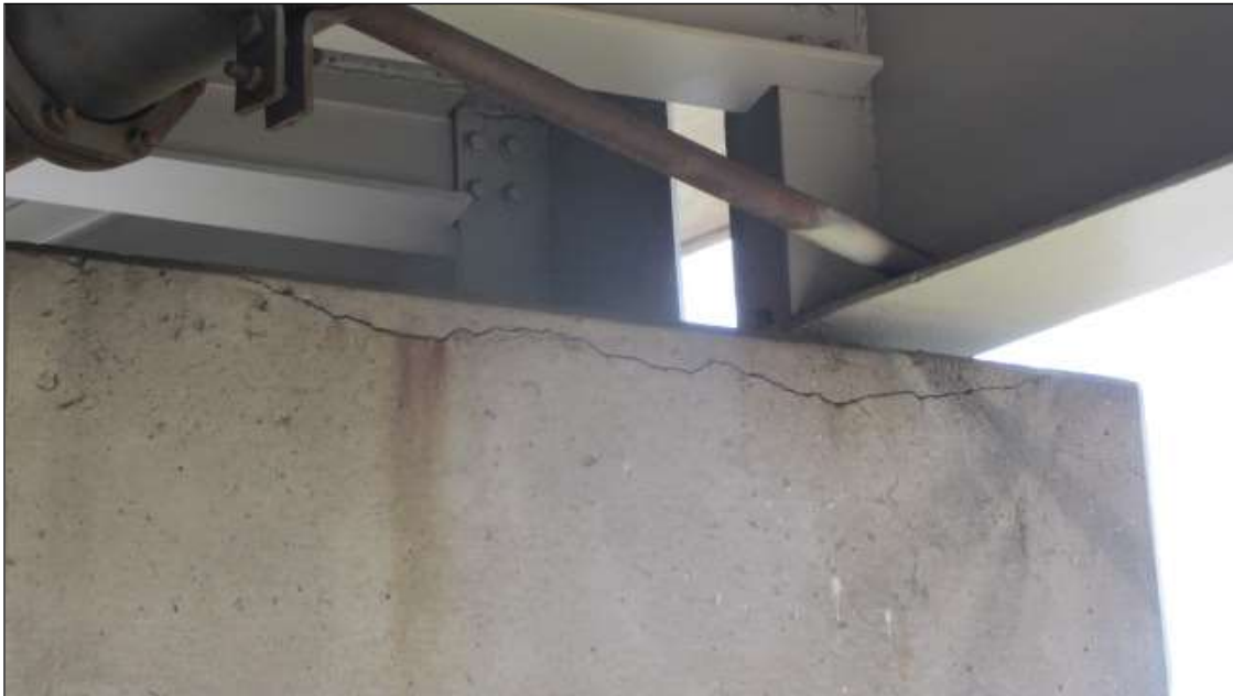
HORIZ. CRACKING ALONG MOST OF THE LENGTH ALONG THE TOP CORNER OF THE EAST FACE OF BENT 3 CAP.
